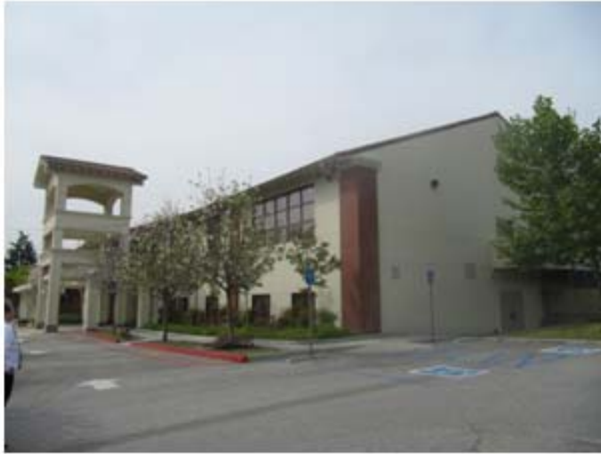
Site Photo 1: East Building
