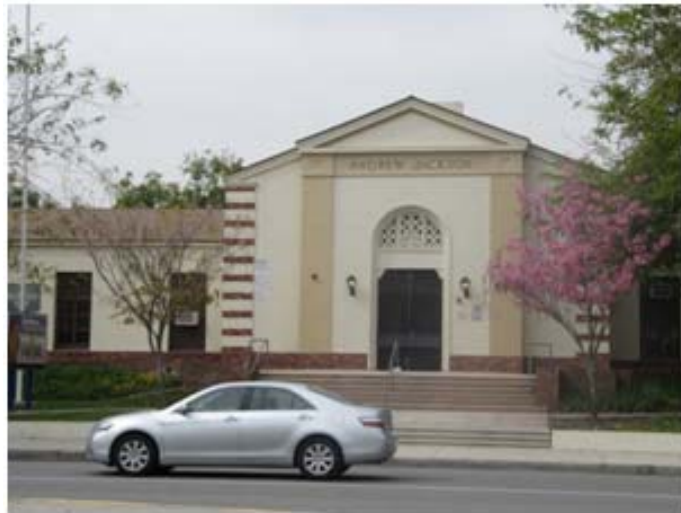
Site Photo 1: School
