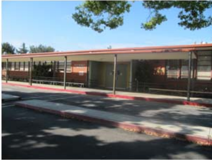
Site Photo 1: School
