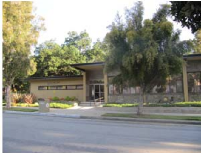
Site Vicinity: Public Library to NW
