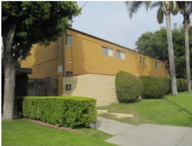
Site Vicinity: Apartments on east
