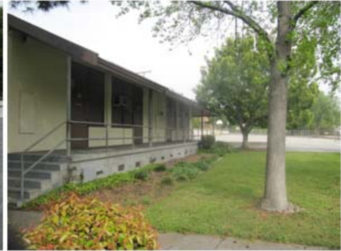
Site Photo 3: West Building
