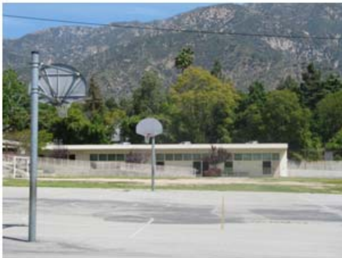
Site Photo 4: New Building
