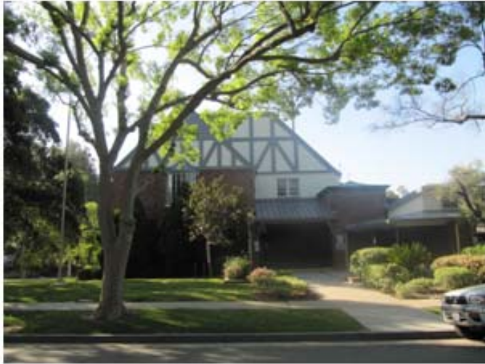
Site Photo 1: School
