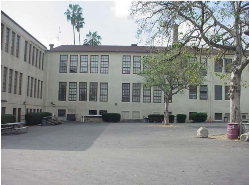
North end, looking West to Main Bldg.
