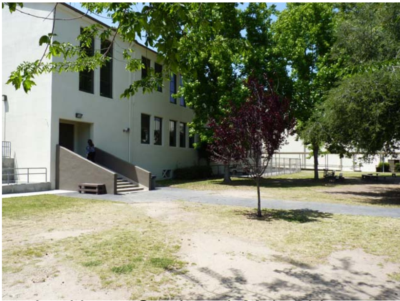
Looking at South end, Main Bldg.
